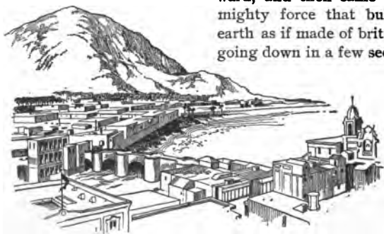
Valparaiso, Destroyed by Earthquake
