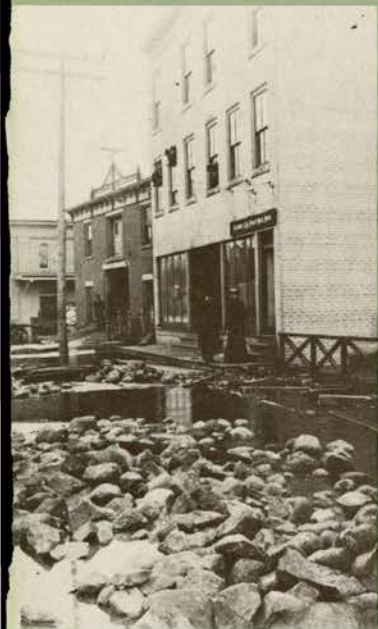
LEFT: Bridge weighted with rocks to prevent it from floating away in the flood
