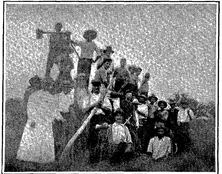
READY FOR WORK AT THE AVONDALE SCHOOL
